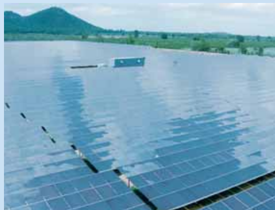
Anwell's first EPC project in Bangkok, Thailand
